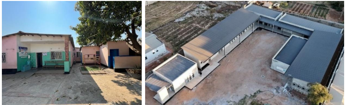
On the left, the existing Little Assisi Day Centre & Special School, with the new, purpose-built school on the right
